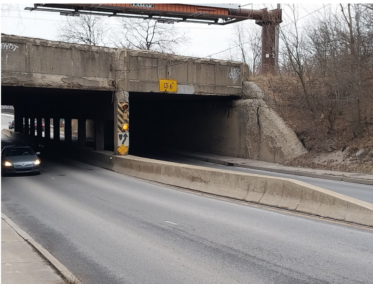
Memphis Avenue Railroad Bridge (Credit: Representative Richard Dell’Aquila)
